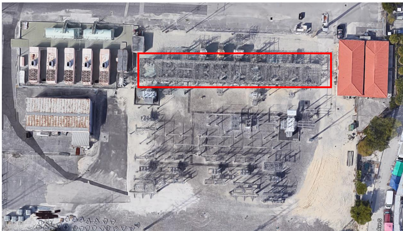
Figure 2: Aerial Image of Main yard substation. Red indicating the 26.4kV bus area.
